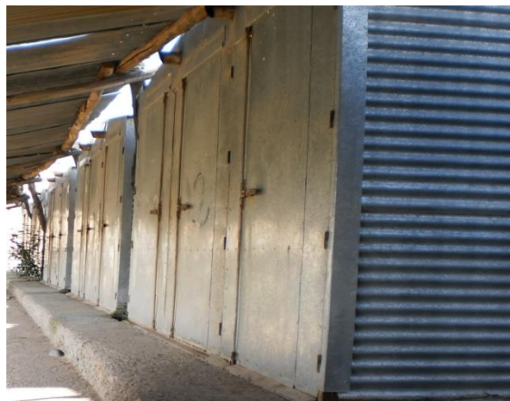
Vista general estufas bulk curing
